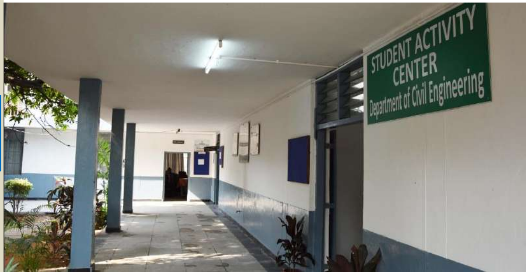
Student Activity Center, CED and relaying of corridor flooring
