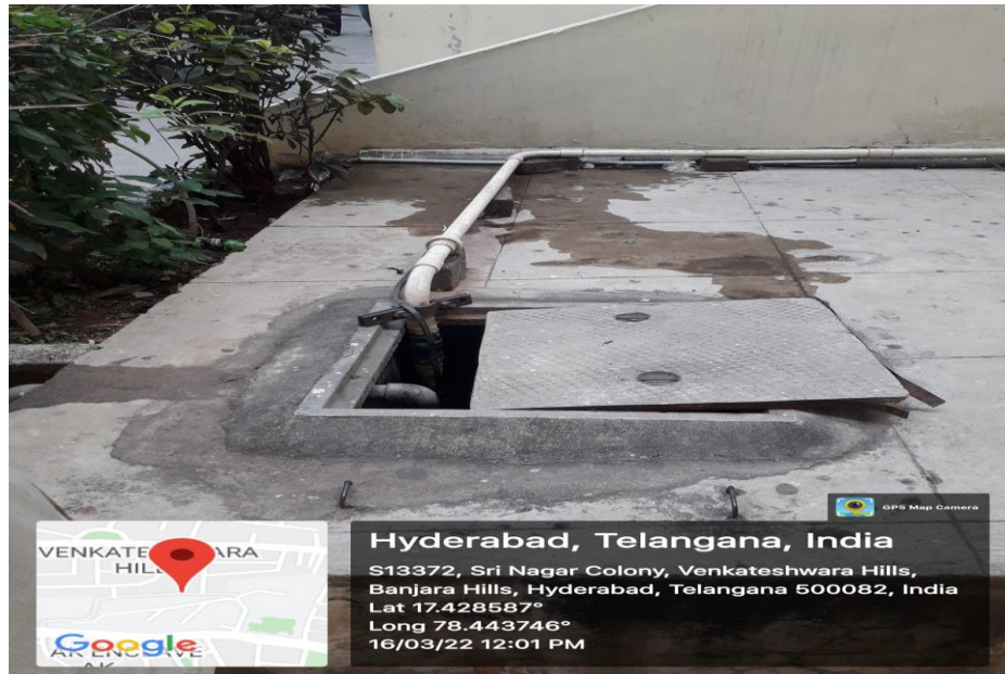
Water Sump and Pipe fitted
