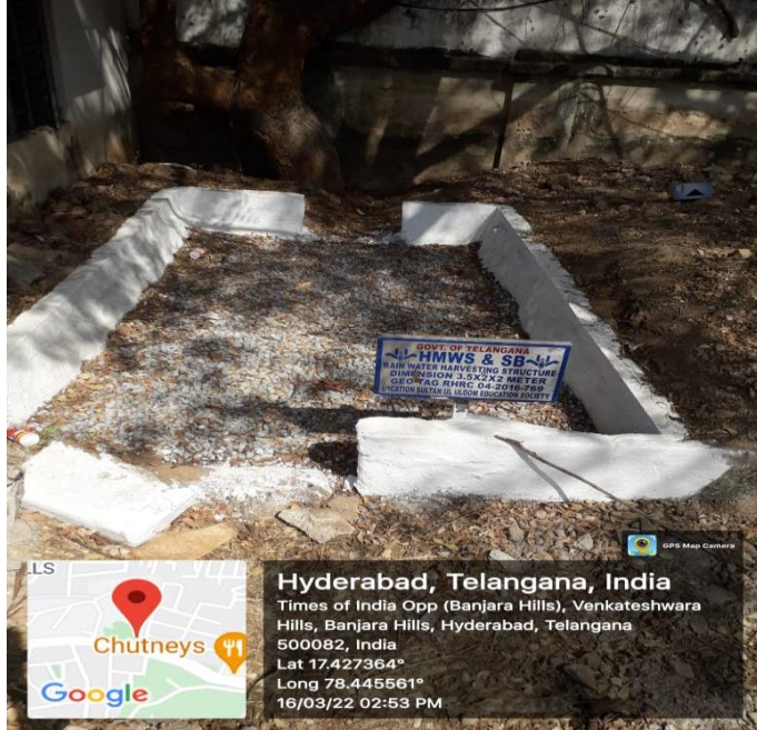
Rain Water Harvesting Pit
