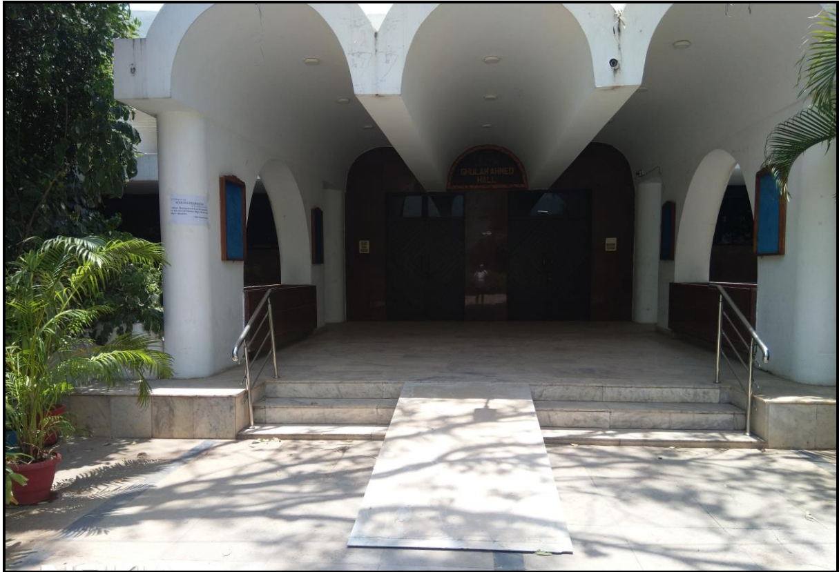
PROVISION OF RAMP AT AUDITORIUM ENTRANCE
