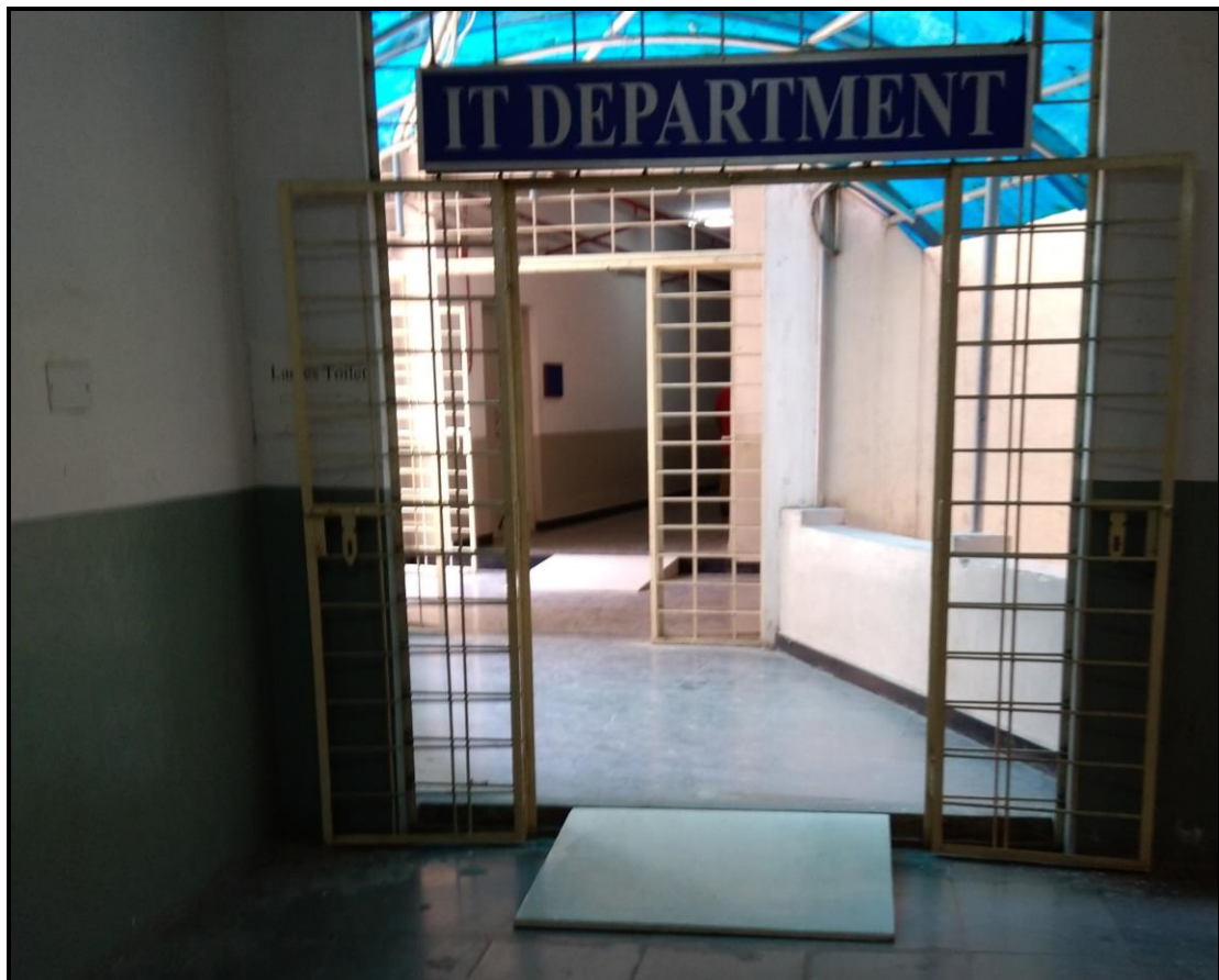
PROVISION OF RAMP AT BLOCK 2 ENTRANCE
