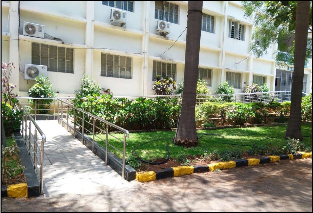
PROVISION OF RAMP CUM RAIL AT BLOCK 1 ENTRANCE
