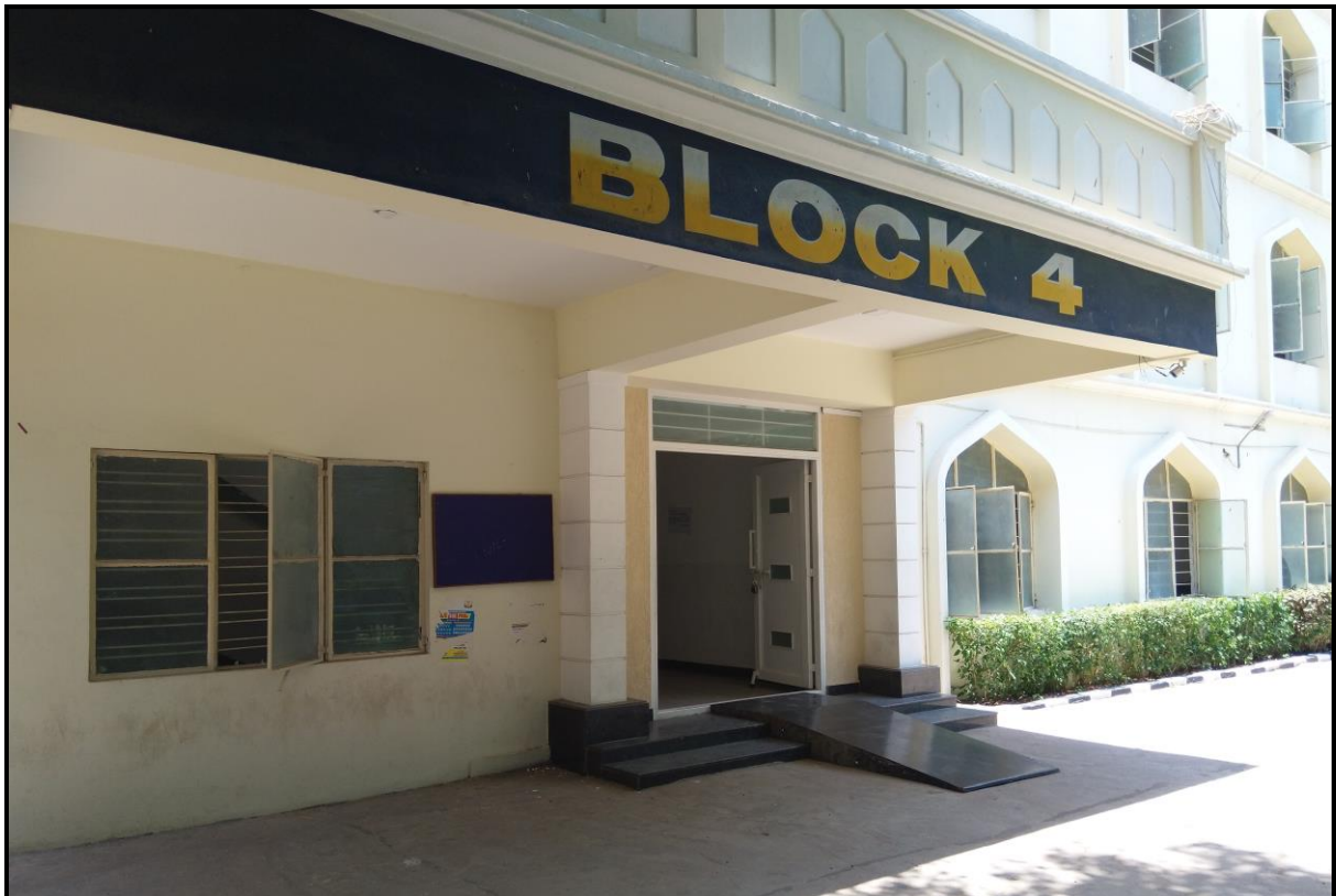
PROVISION OF RAMP AT BLOCK 4 ENTRANCE
