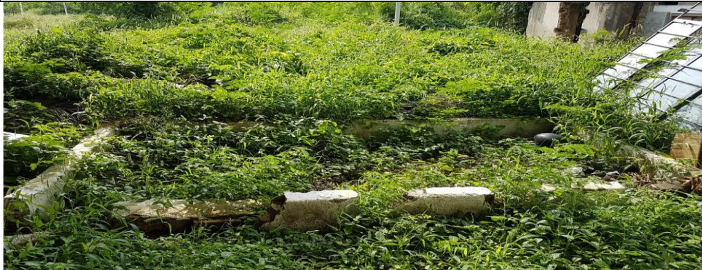
Fig: Rainwater harvesting structure inside the college campus
